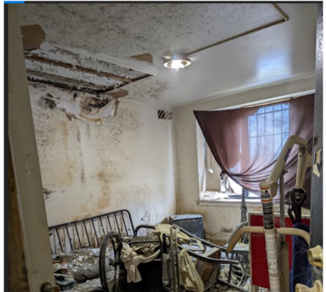
Photos: Mold/mildew and moss growing in a vacant unit that was discovered with an active leak (top left and right). Mold/Mildew on walls and floor (left) and wall and ceiling (right) in vacant/abandoned units. These units represent the most extreme examples encountered.
