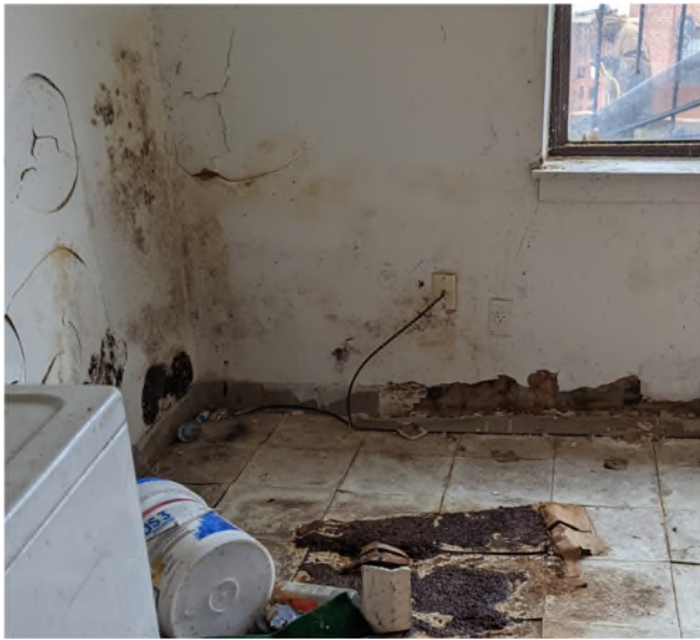
Photos: Mold/mildew and moss growing in a vacant unit that was discovered with an active leak (top left and right). Mold/Mildew on walls and floor (left) and wall and ceiling (right) in vacant/abandoned units. These units represent the most extreme examples encountered.
